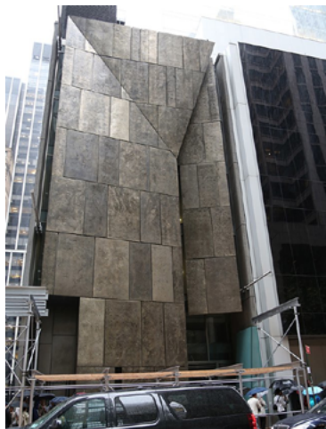
Scaffolding goes up to take down the Folk Art facade.
