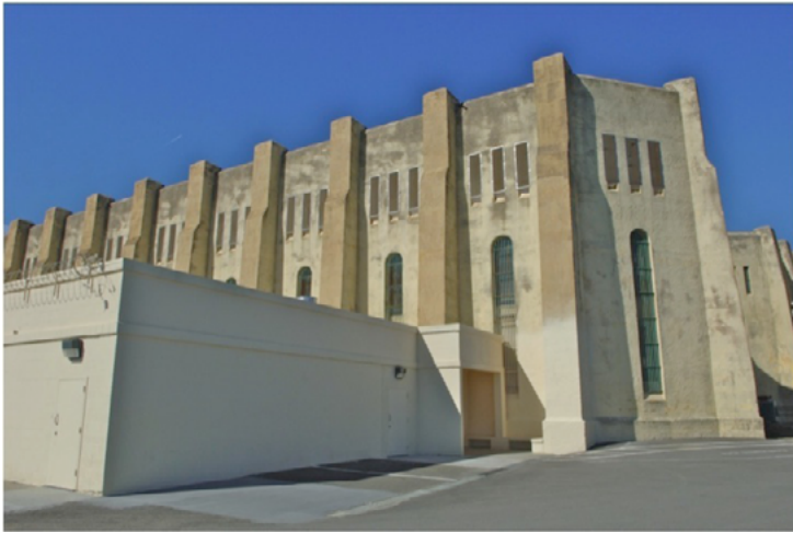
The Lethal Injection Facility is the windowless box adjacent to the older, still functional cell block. The CMU exterior walls predate the interior renovations for the new death chamber.
