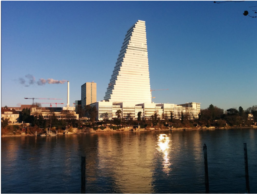
Roche Building 1. Photograph by the author.
