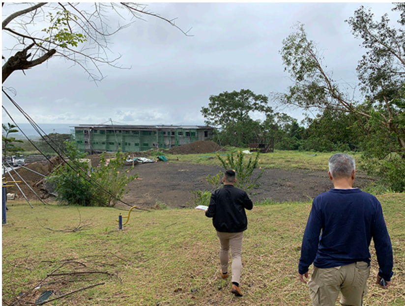
The Horizon Condominiums under construction at Tagaytay Highlands. Photograph by the author.
