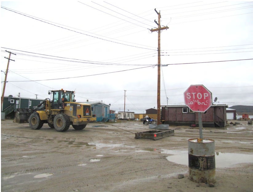
Flattening of the road in Kangiqstugaapik, Baffin Island, Nunavut. Courtesy of the author.
