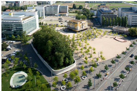
Leutschenpark today, with the wall encasing the former bullet trap. The structure was nicknamed the "plant pot" by the architects and the municipality. Courtesy of the architectural history archive of Zurich.
