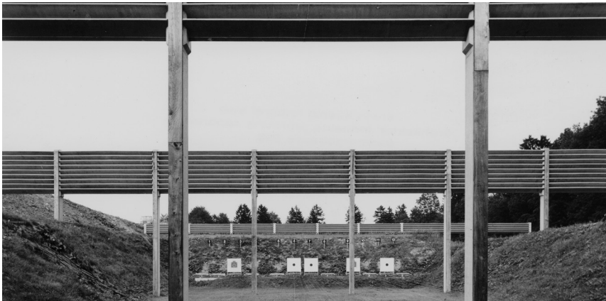
An earth wall used as bullet trap at the Allmend Fluntern shooting range, which was in operation from 1971–2005. Courtesy of Architectural history archive of Zurich.
