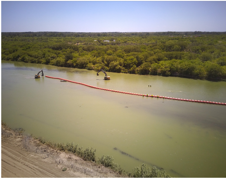
Construction of a floating barrier in the Rio Grande near Eagle Pass, Texas, July 17, 2023. Courtesy of Wikimedia Commons.
