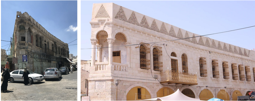
Left: The museum in 2019 before its renovation. Courtesy of the author. Right: The museum in 2022 after its renovation. Courtesy of the Hebron Rehabilitation Committee.
