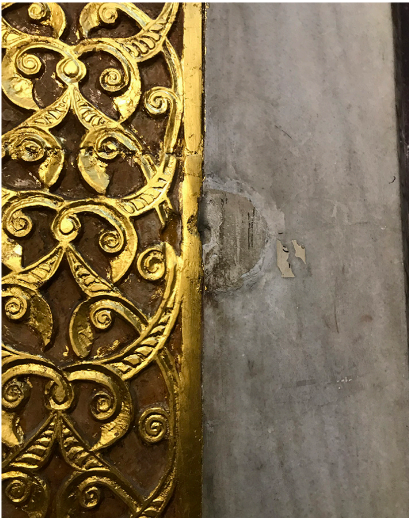
A patched-up bullet hole next to the newly regilded ornamentation at Al-Ishaqeyyah Mosque, July 17, 2019. Courtesy of the author.
